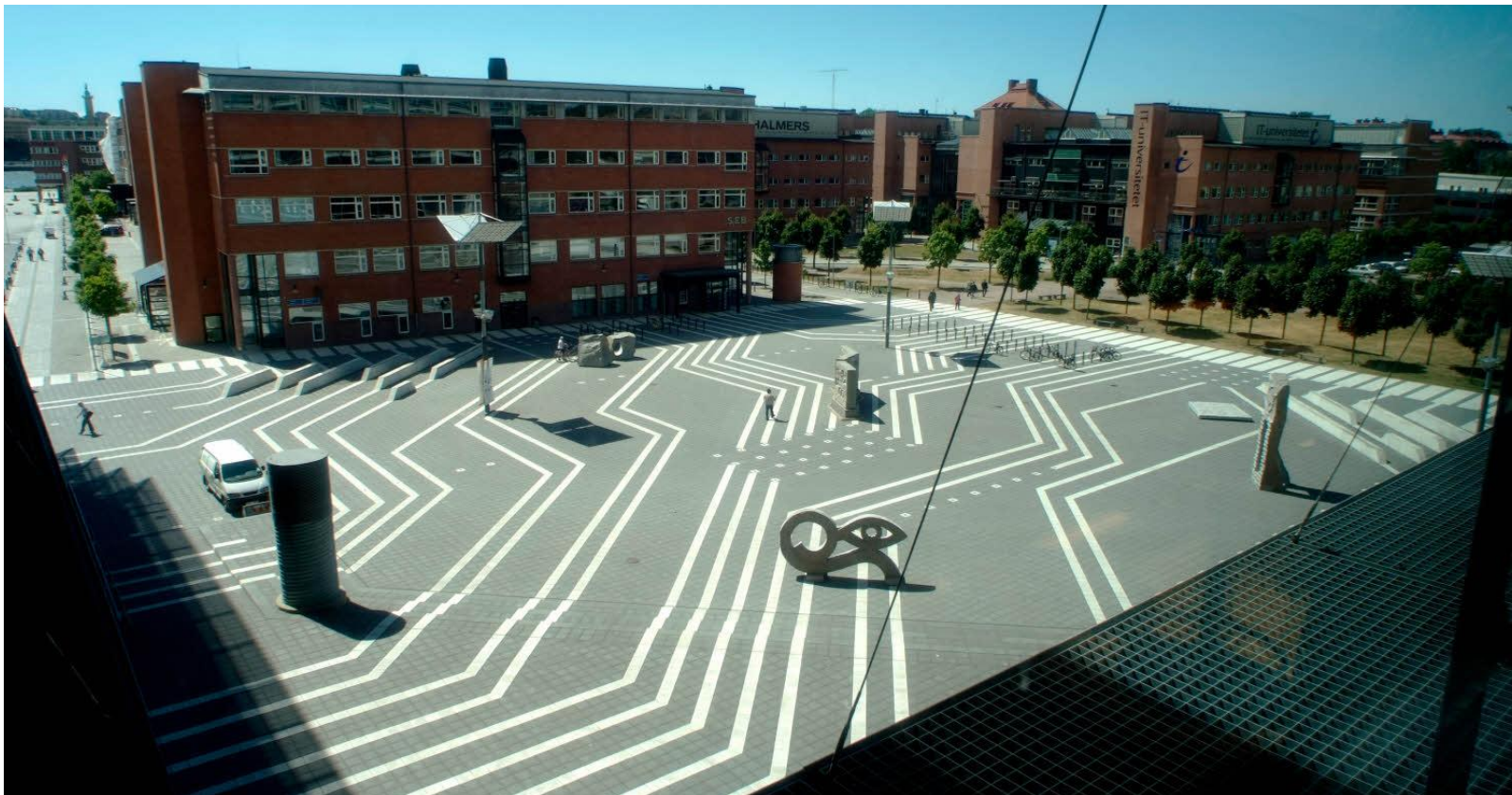
The ground slab Superplattan at Lindholmsplatsen i Göteborg.
