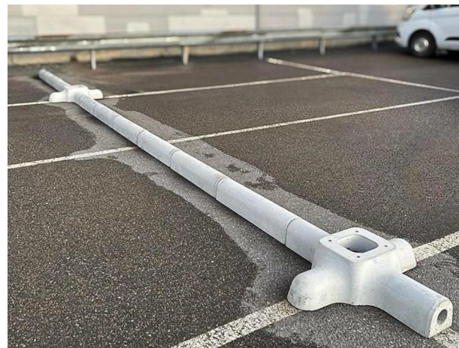
Hollow cable stones are used to lay cables across a parking area to charging stations for electric vehicles.
