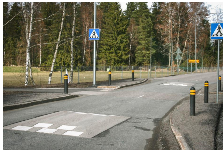
Speed cushions at a pedestrian crosswalk.
