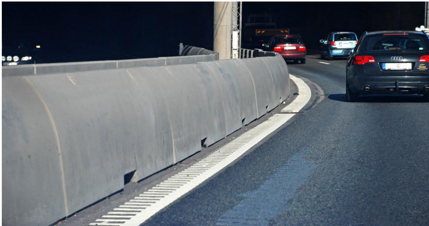
The road barrier element Linebloc separate the lanes.
