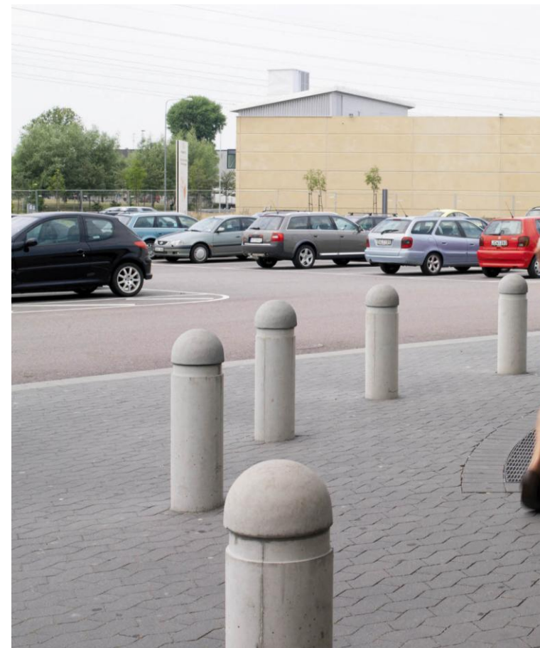
Bollards Freja protecting a shop entrance.
