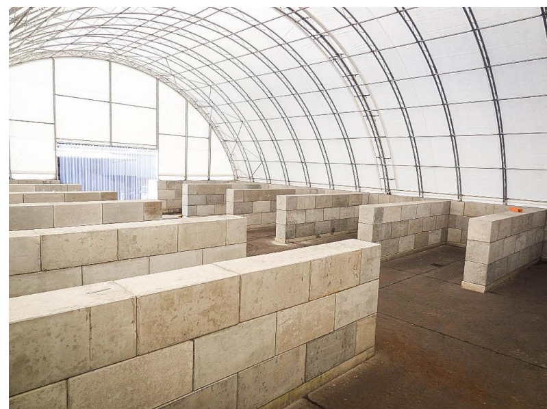
Flexiblock used to build loading pockets.
