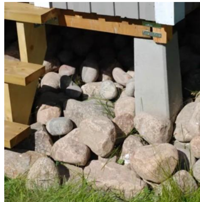
A plinth used to anchor a small wooden structure.
