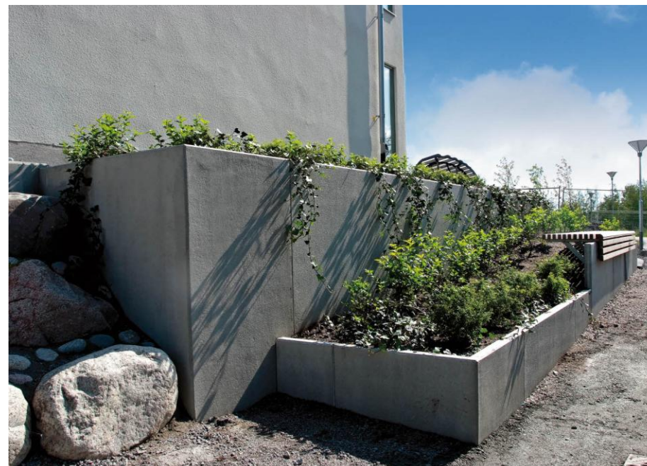
Retaining walls used to create flower beds.
