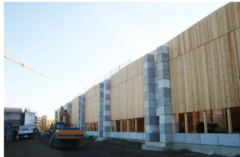
Flexiblock integrated into a house construction.
