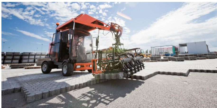
Machine laying of Hexasten paving stones in Umeå speeds up the construction work.
