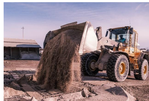
A wheel loader pours aggregate through a grid onto the conveyor belt that will take it to the silo.
