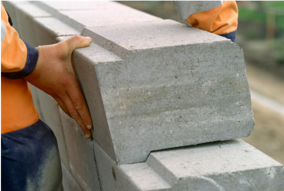
Retaining wall blocks.
