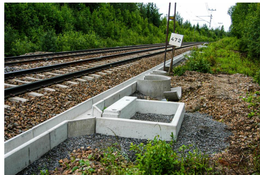
Foundation for signal cabinet and wells for wires.
