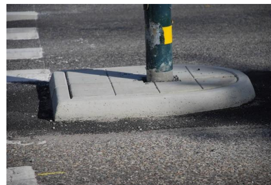
The kerbstones G-Refugen at a traffic island.
