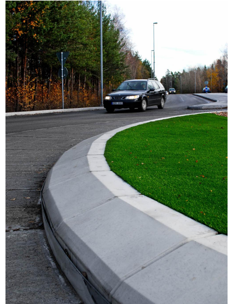
Kerbstones in a roundabout.
