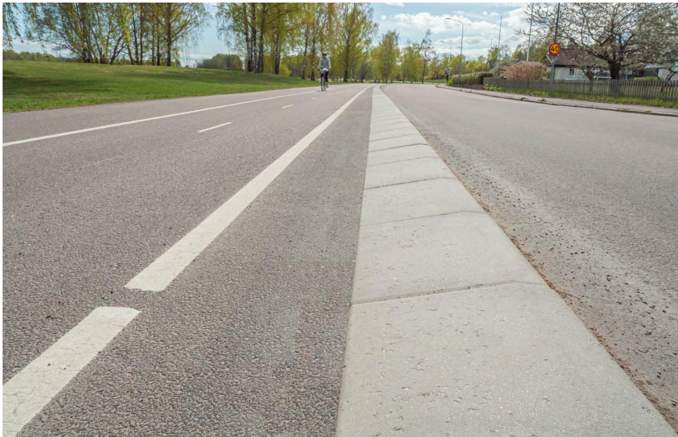
The kerbstones GCM-stöd separates a cycle lane from the road.
