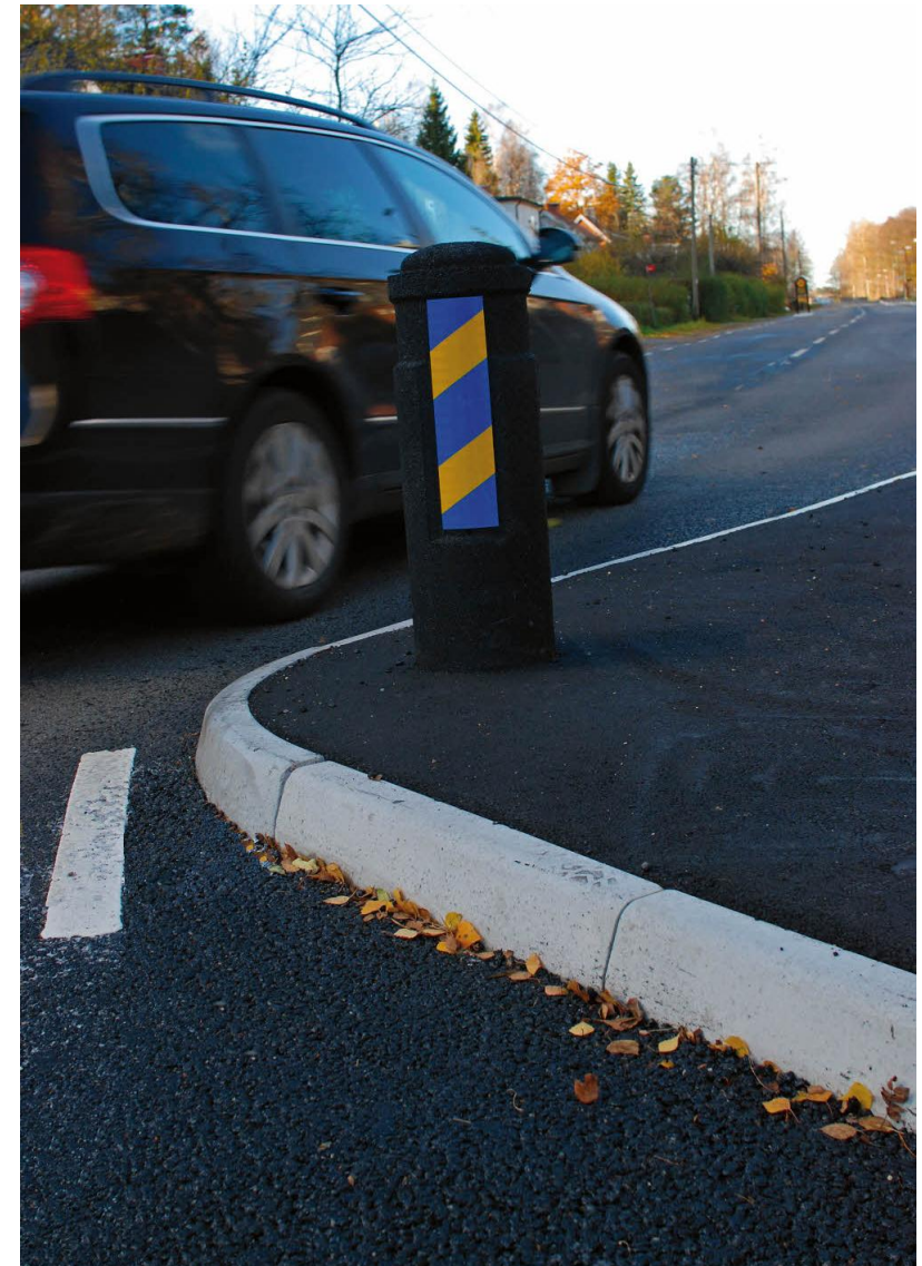
Kerbstones for streets at a pavement.
