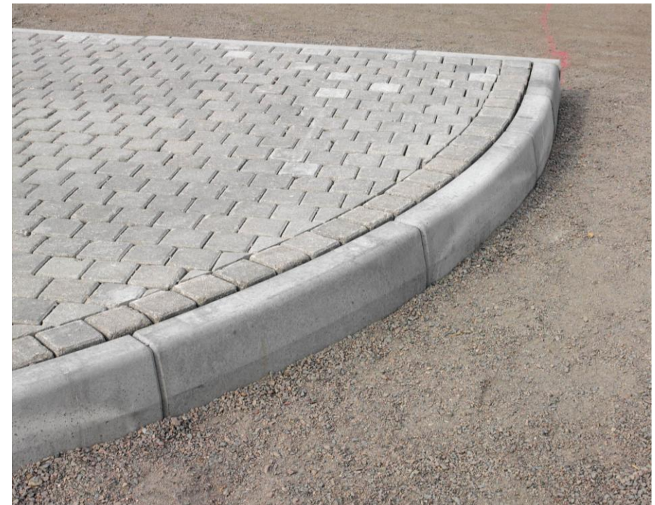
Kerbstones for streets recently installed at a construction site.
